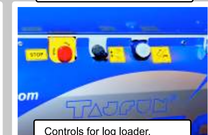
Controls for log loader, conveyor belt; STOP function
